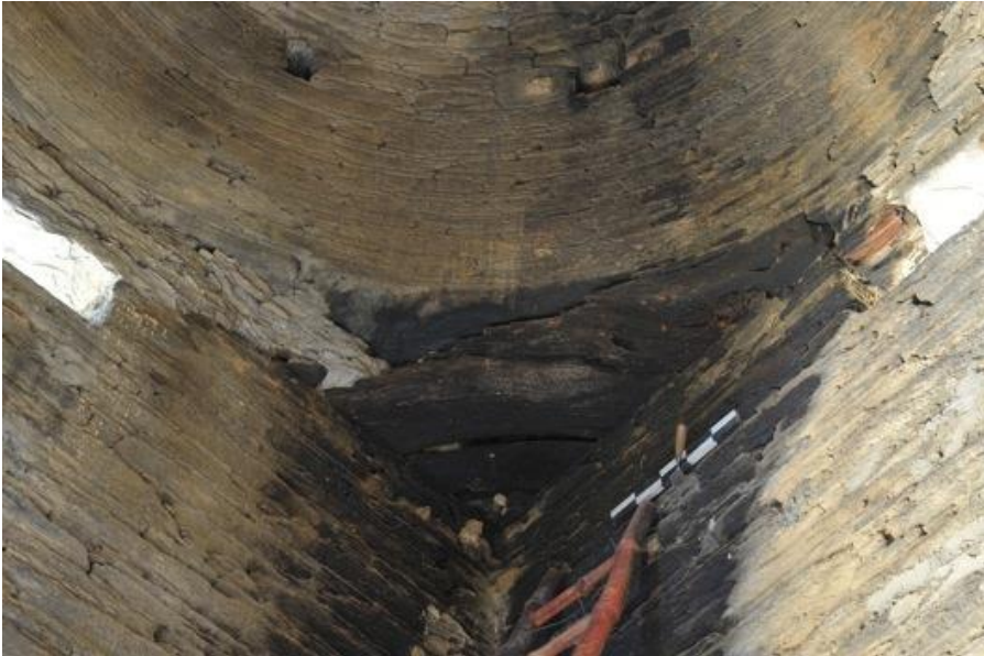
Fig. 63 - The three SE corner beams and S clerestory lintel (Photo by EL).
