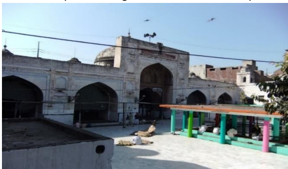
Fig. 3 Ugly electricity wires; edition of modern shade in bright colours and floor of the courtyard paved with modern tiles
