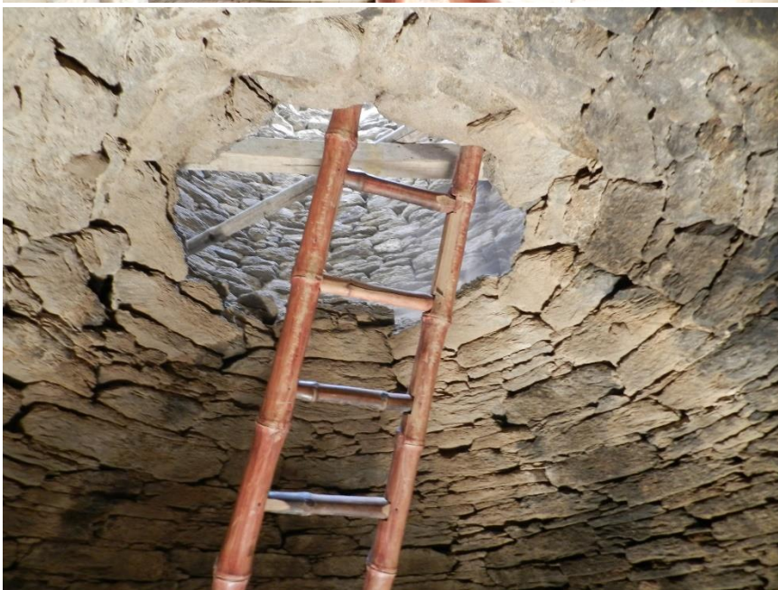
Figs 9-10 - Conservation in progress (below: a detail of the double domes) (Photos by FM).
